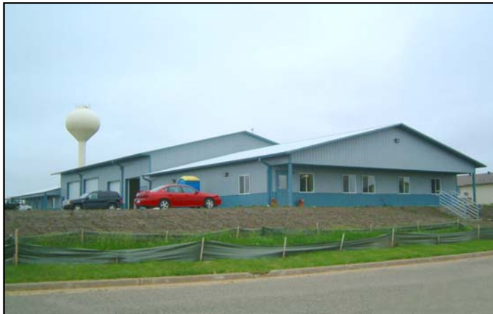
The Police Department is located on the right side of the building, EMS is on the left side, and vehicle garages are in the center.
